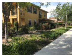
Recently approved area renovations begin in March along Towngate.
